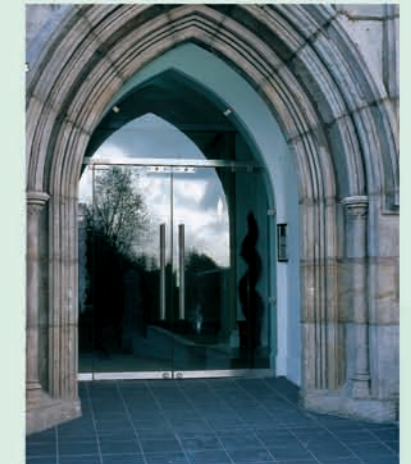
Church Apartments, Manchester
